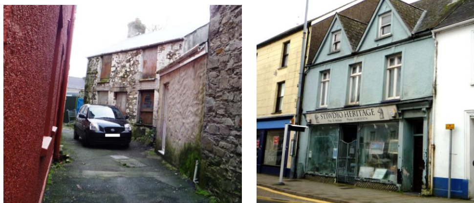
Properties requiring repair or renovation (23.11.15)
