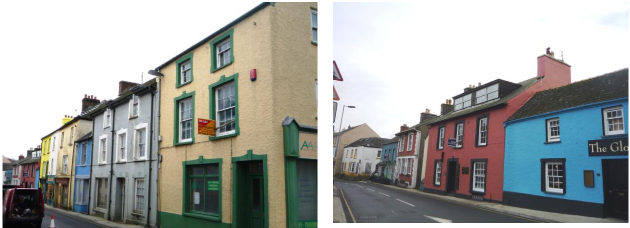
Various Properties (Even Nos.) at Main Street (23.11.2015)
