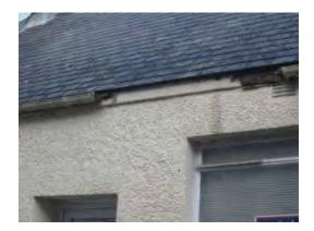
Missing and damaged gutters should be repaired, to avoid water penetration and damage to buildings (above right). The clumsy design of rain water goods, and poor quality materials have a negative impact on the building's elevation (above left).
