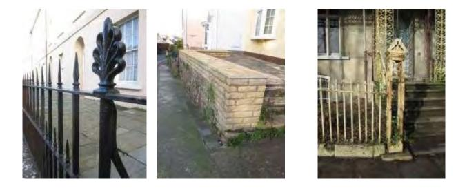
Repairs or replacement should always be in the same material as the original. For example, the use of brick to repair a stone boundary wall (above centre) should be avoided.
