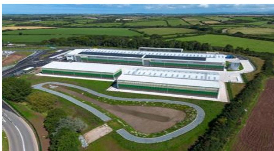
Image 1: Pembrokeshire Eco Park – Waste Transfer Facility.
