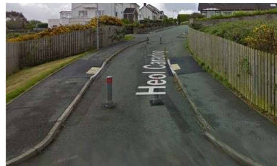
Existing barriers to the bus service on Heol Glyndwr and Heol Caradog
