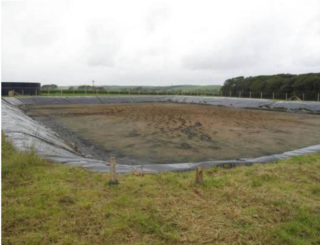
Earth bank lined slurry lagoon
